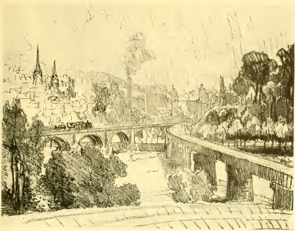
THE RAILROAD BRIDGES AT FALLS OF SCHUYLKILL
